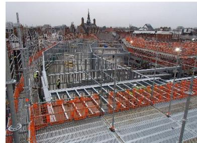
This is a view of the roof trusses on the Anchor Unit next to the Redan Public House. This building has three pitched roofs, each made up of sixty trusses. The roofs will be clad with natural slates. Three feature brick gables face Peach Street and the Piazza. The plant space has been incorporated into the roof structure. Brickwork is progressing from ground to first floor level, English Bond is being used on this building.
