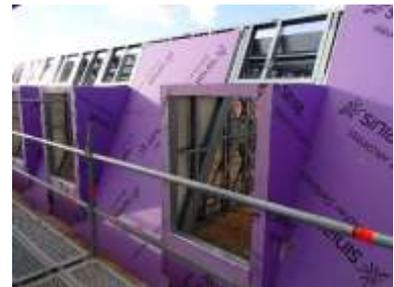
This also forms the primary air seal to the apartments. The mansard and dormers will be clad with a zinc metal rainscreen to provide the final weatherproof layer and architectural feature. The second photo shows the roof construction over two of the apartments that face onto the new piazza. The first layer of waterproof membrane has just been laid. This will be covered with a layer of insulation and capped off with the final single ply waterproof membrane.
