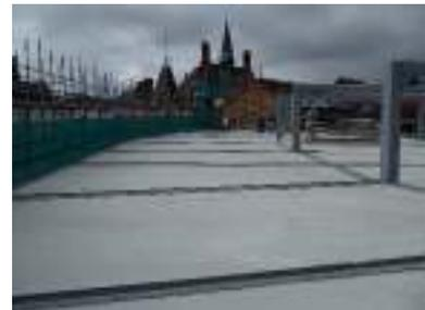
Here's the same view at ground floor level from the new arcade, looking back towards Costa. The 5 new shop units will face onto Peach Street. The edge shuttering is in position, the drainage and service ducts have been installed, the insulation and reinforcement is being laid ahead of the concrete pour planned for later this week. The shop units are to be constructed as shell and core, complete with double glazed shop fronts ready for the tenants to fit out.
